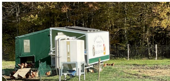
Power supply of a mobile chicken shed
