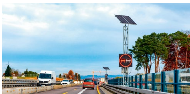
LED road sign
